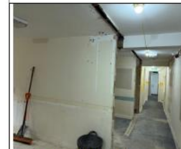
Changing rooms demolition in progress
