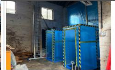
Asbestos removal to White Barn Anex
