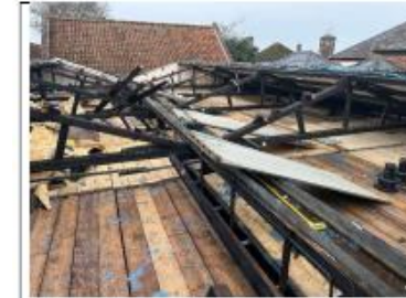
Shakespeare's Barn roof removal
