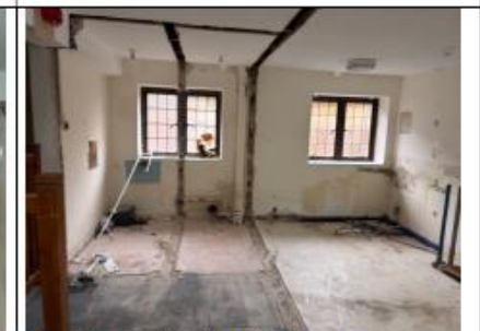
Changing room WC demolition in progress
